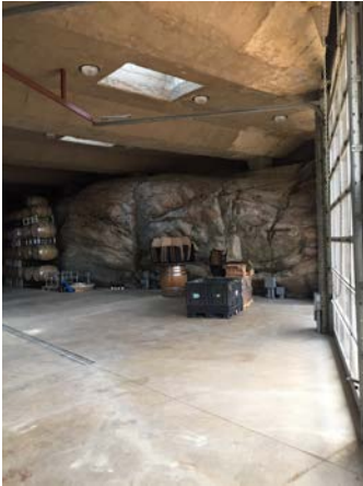
Inside the natural fault, now Pentâge Winery's cellar
